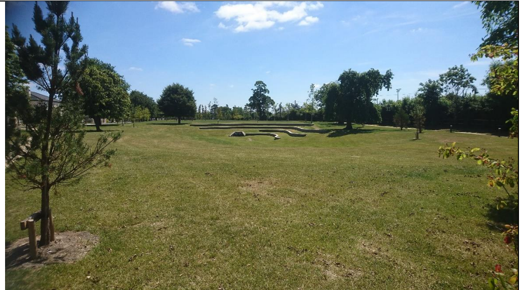
Fig.1 An example of a useable detention basin as amenity space in Diswilltown Manor Scheme, Castleknock, Fingal.
